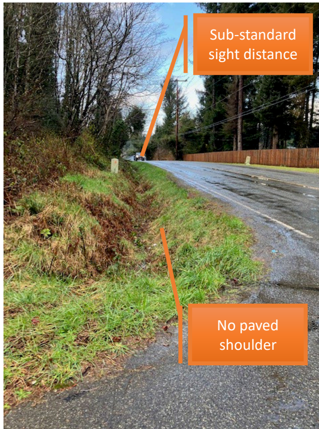
Figure 3: Elk Valley Road at Cassel Lane, looking south
