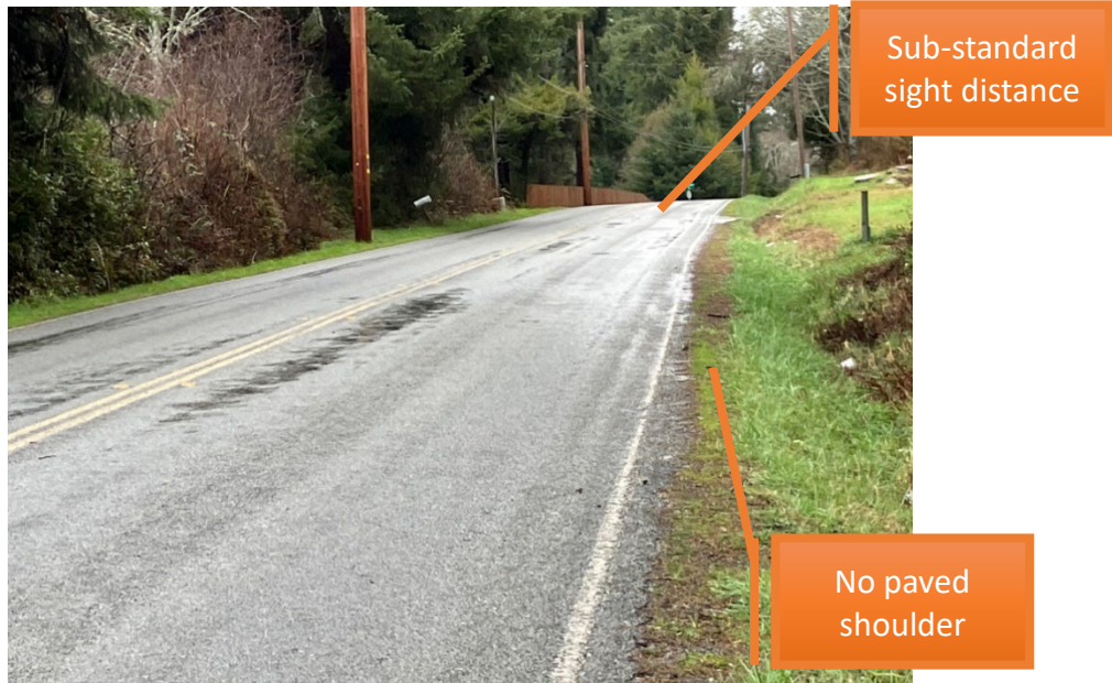
Figure 2: Elk Valley Road at New Hope Lane, looking north
