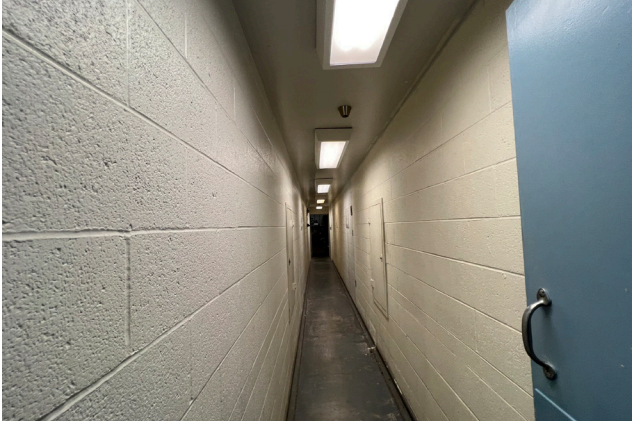
Corridor between Pod D & Pod E
