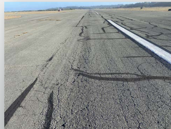
Runway 18-36 Cracking
