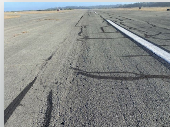
Runway 18-36 Cracking
