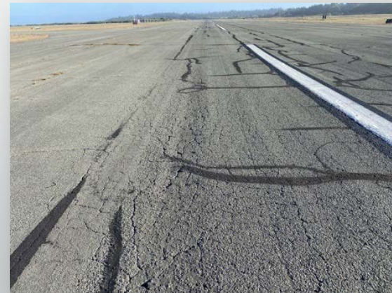
Runway 18-36 Cracking
