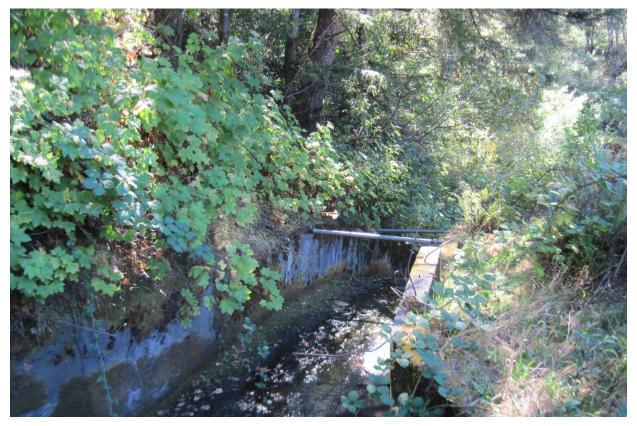
Photo 12B. Tilting and braced spillway walls looking southeast.
