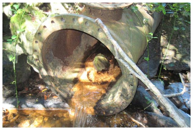
Photo 8B. Water flowing from the discharge pipe at the toe of the dam.
