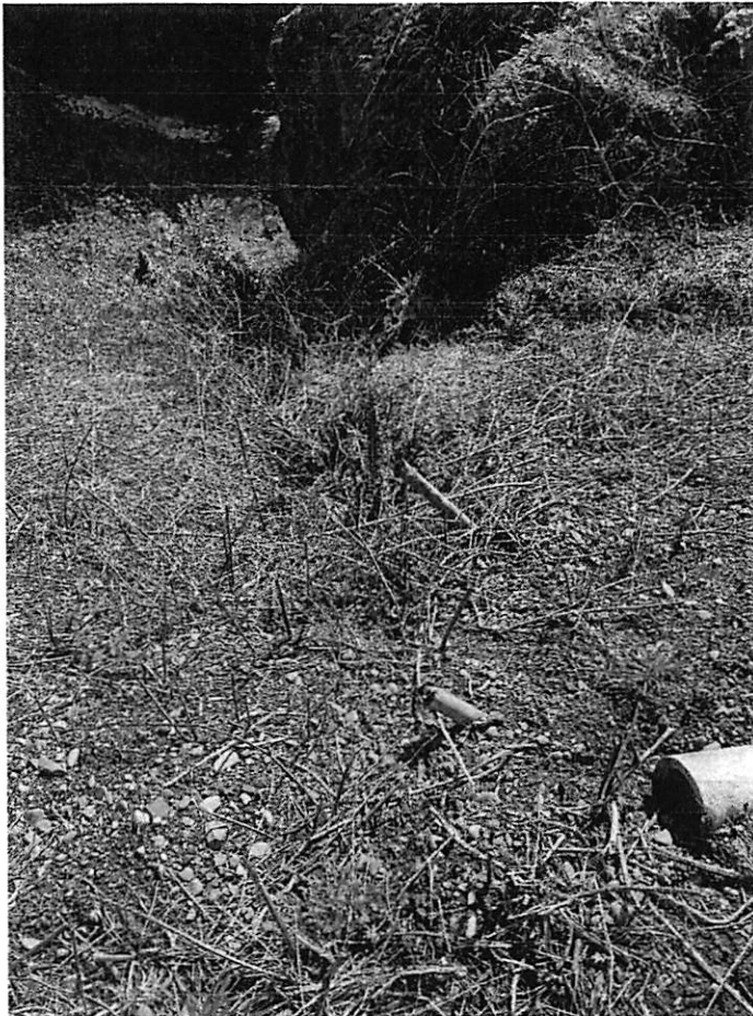
Erosion likely caused by dam overtopping in the past
