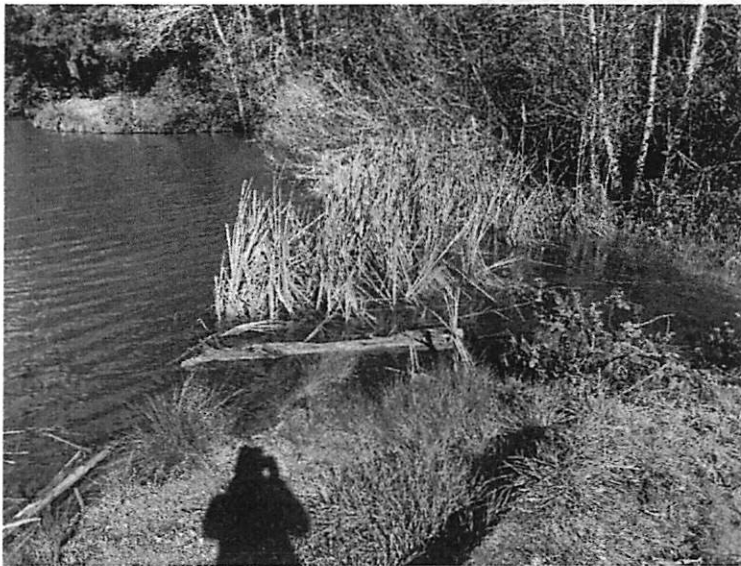
Spillway approach channel overgrown with Cattails
