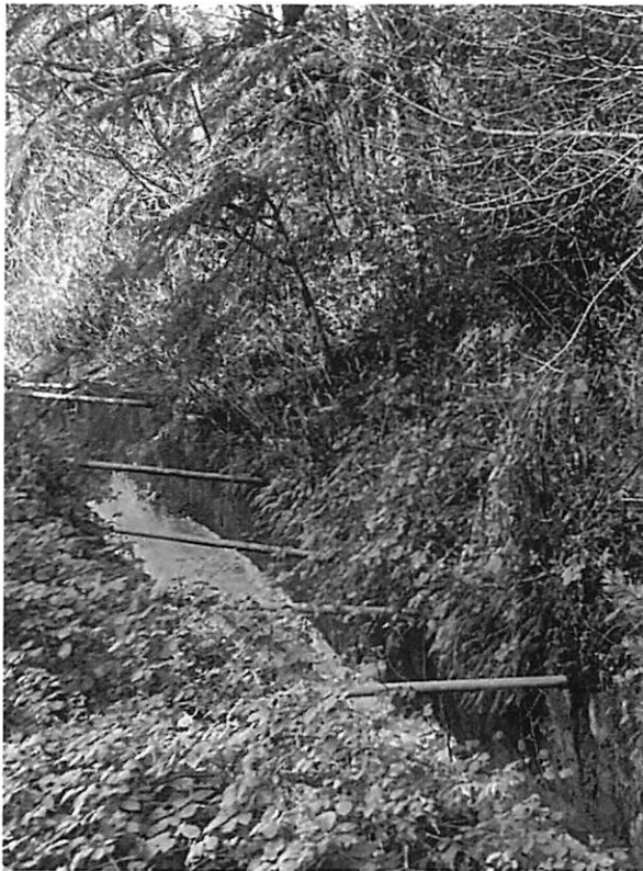
Concrete-lined spillway deteriorating from uphill slope movement
