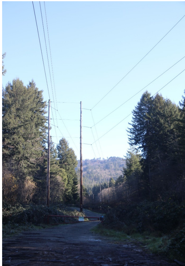
Figure 3. Two parallel 115-kV transmission lines run northeast from Crescent City toward Grants Pass where they connect to 500-kV lines.
