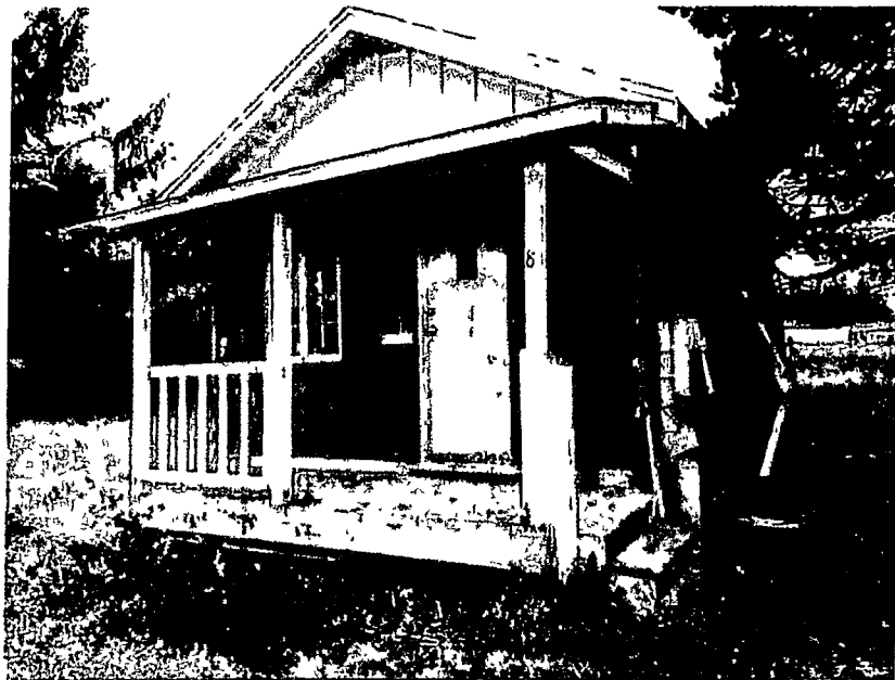
1600 Northcrest Drive Photo of the Existing & Restored Framing
